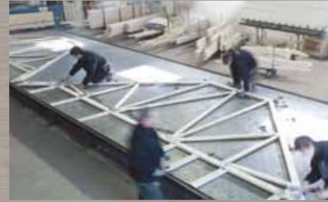
Manufacturing of roof trusses
